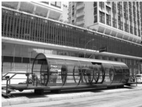
Brazil's BRT boarding islands provide for fare collection and a platform level with the bus, speeding both boarding and deboarding
