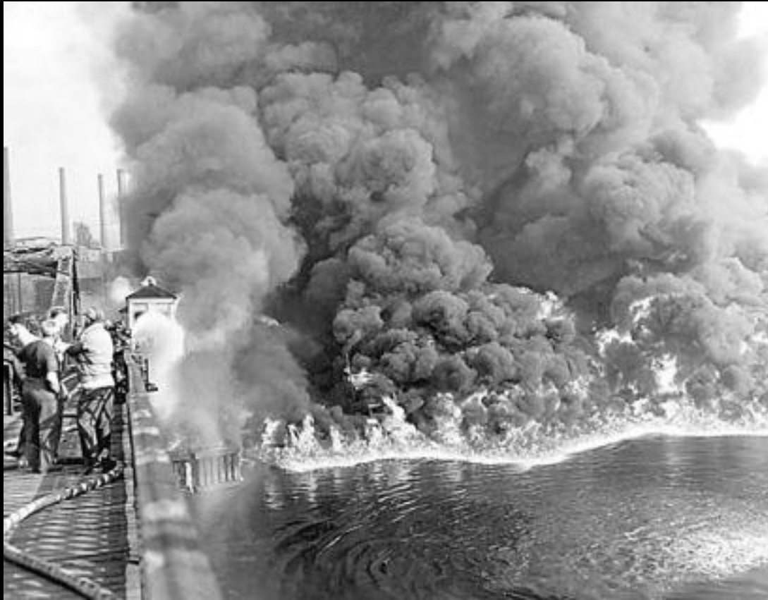
Cuyahoga River Fire – Cleveland Ohio USA – November 3, 1952
